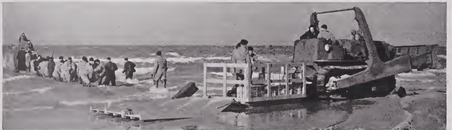
FIGURE 99. Men carry cargo from LCV to waiting bulldozer and sled.
